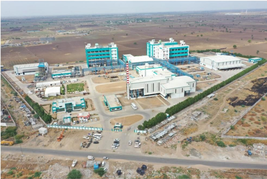
Newly constructed Agrochemical manufacturing plant by NBR in India
