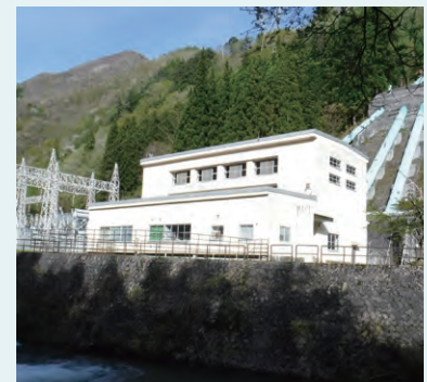
▲ Kuzuyama Power Station
