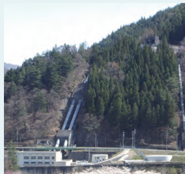
▲ Miza Power Station
