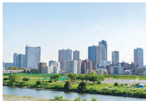
▲ Industrial water treated with wastewater (illustration purposes only)
